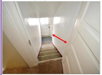
15. Stairs to the Basement will need to have a hand rail installed as per UBC codes.
