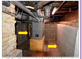
Ruud furnace was installed & elevated correctly within a dug-out area in Basement and has been installed with new poured concrete retaining walls.
