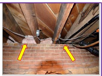
20. Brick stem walls and heavy timber joists are not anchored to the brick opposing any seismic activity that may need remedies by an Engineer.
