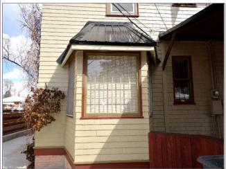
5. Typical example of the "black" Propanel roof systems installed on building "pop-out" room are in Satisfactory Condition.
