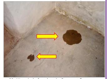
30. Water leaks found on the Basement floor.
