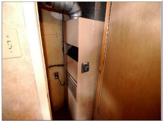
28. Ruud Furnace found on the Second Floor has minimal access within a tiny closet with the Richmond H<sub>2</sub>O heater. Verify with a plumber.
