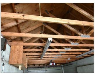
10. Typical engineered trusses built over the Tandem Garage were properly executed and sound.
