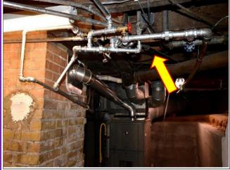
17. Galvanize pipe & valves found on the ceiling in the Basement have been painted with silver paint and are in Satisfactory Condition.
