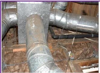
13. Heating ducts found in the Attic have been properly installed and joints were taped with duct and silver tape as per UBC codes.
