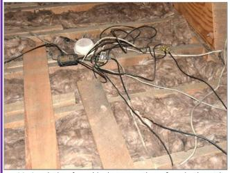
Insulation found in-between the rafters in the attic are in Satisfactory Condition. Messy wires will need to be straightened out.
