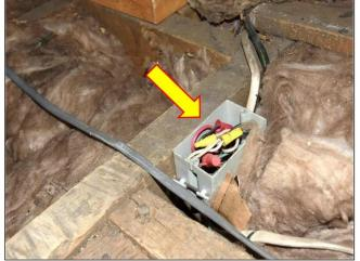
12. Open electrical boxes will need to have cover plates provided to avoid electrical fire hazards.
