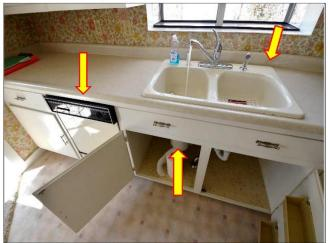
39. An Air Gab is needs on the countertop to provide proper vacuum break on the sink's trap due to having both a dishwasher and waste disposal.
