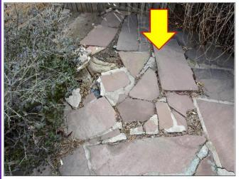
53. Some of the flagstone on the property is dislodged will need resetting and reappointments with the joints and cement grouting.
