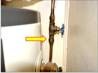
26. Shut-off valve to  $H_2O$  heater has a slow leak running to the basement floor and must be fixed to prevent further damages.
