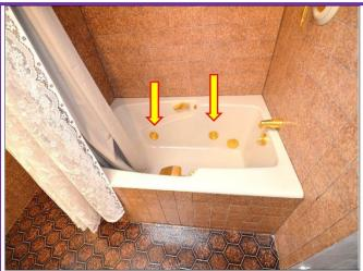
49. Guest Bathroom's bathtub on the Second floor with tile walls and vinyl floor has non-working air jets, "whirlpool" are not working, needs repairing.
