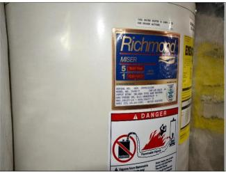
27. Richmond H<sub>2</sub>O heater found on the Second Floor has minimal access within a tiny closet with the Ruud furnace. Verify with a Licensed plumber.
