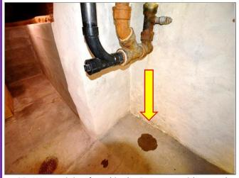
29. Waste piping found in the Basement with recently installed plastic ABS pipes is leaking and this needs to be fixed by a Licensed plumber
