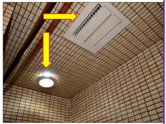
46. Master Suite bathroom's fan is not working and light trim needs to be reset. Tile ceiling and walls are in Satisfactory Condition.
