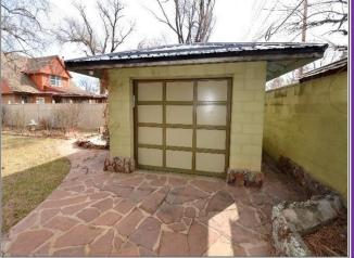
6. Auxiliary Building made of CMU block walls is Auxiliary Building. Flagstone needs some masonry attention.
