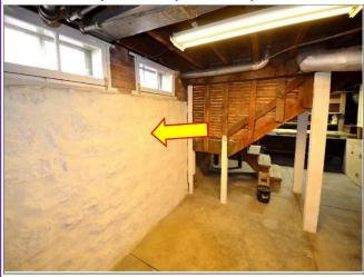
21. Painted rock & mortar stem walls were found in the Basement and installed correctly with poured concrete floors.
