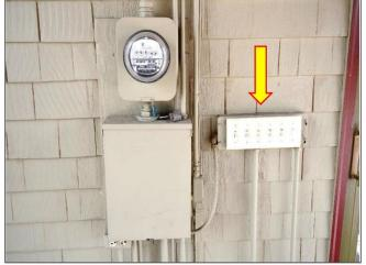
24. Plastic switch cover plate covering 6-gang switches is not correct for exterior uses. Electrician shall provide a correct 6-gang metal cover plate.
