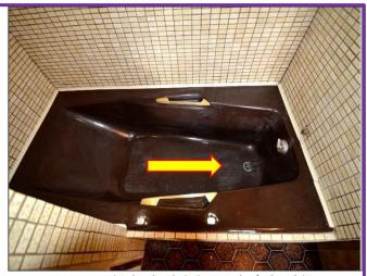
50. Master Suite bathtub is in need of plumbing repairs, especially around the drain stopper.
