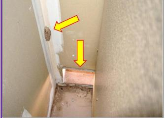
1. Combustible Air Vent to the Mechanical Closet has a problem with the lack of an insect screen to prevent wasp and wasp nests from entering the closet.
