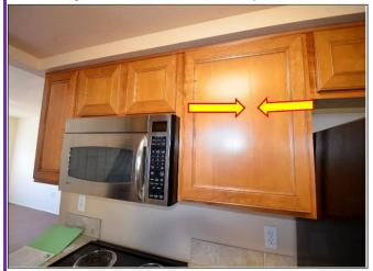
5. Kitchen Cabinet door is blistered and will need to be refinished with proper cabinet making detailing.
