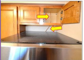
3. <sup>1</sup>/<sub>4</sub>" copper tubing from the Mechanical closet routed through the cabinet and behind the Refrigerator for the icemaker to operate.
