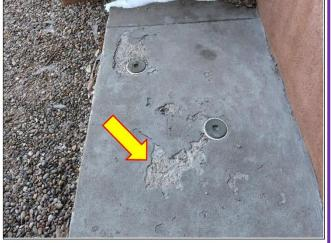
12. Typical concrete sidewalk that will need to be resurfaced due to spading and erosion.
