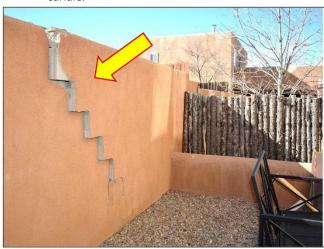
10. Apartment Two's Patio wall on backyard that is in failure.
