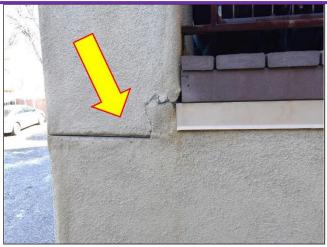
7. Flashing failures on all of the Balcony decks that will need to be repaired and re-stucco.
