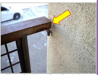
28. Most of the Balcony railings will need to be secured to the wall with solid steel spacers.
