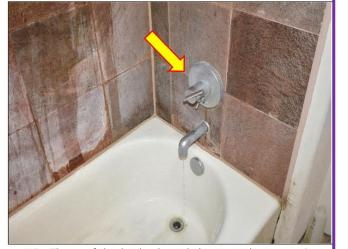
18. Three of the bathtub and shower valves were in Poor Condition and the diverter valves were not properly working and will need to be replaced.
