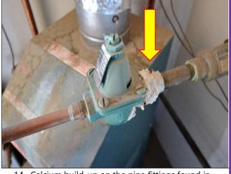
14. Calcium build-up on the pipe fittings found in most of the Mechanical closets that will need to be cleaned with solvents.
