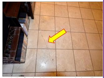
16. First floor level showing many cracks that will need profession attention to remove and replace with a tile isolation membrane.
