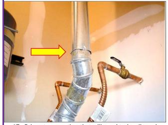
17. Exhaust connection that will need to be silvered taped to seal properly.
