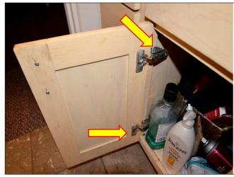
22. All cabinet doors on the Kitchen and Vanity cabinets will need to have the hinges exchanged for the proper euro stiles type of hinges.
