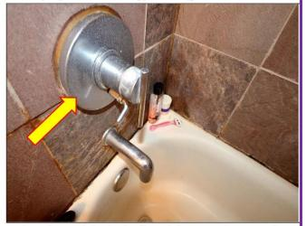
24. Three of the bathtub and shower valves were in Poor Condition and the surround tile walls will need to be cleaned and the caulked to properly seal.
