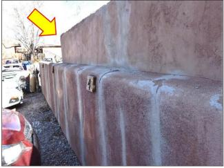
Parking lot wall that was not repaired correctly and will need patching and re-stucco with color coat.
