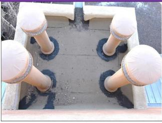
Upper Mechanical shafts rooftops that are in Good Condition with roof jacks and drainage to canale.
