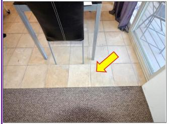
23. Second floor level is also showing cracking on the cermeric tile floors and will need to be removed and replaced with a tile isolation membrane.
