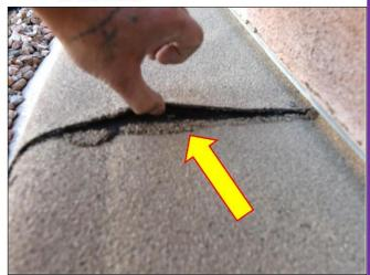
Neighbor's building is showing some Torch-down failures on an overlap that could impact the Inspected "810" Building.
