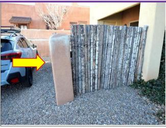
20. CMU block column is badly leaning on Apartment One's Patio with the possibility that the cause is due to Storm drainage equipment.
