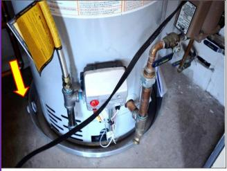
15. Five of the safety pans under the H<sub>2</sub>O heaters will need a drainpipe and routed to an outside wall for proper drainage.
