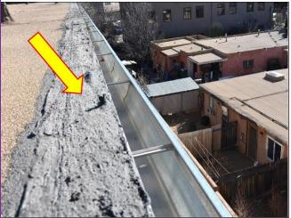
Drainage edge to Gutter is in rough shape with nails sticking up and will need serious repairs.
