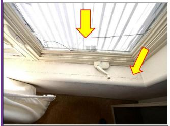
21. Bedroom window on Apartment Three is broken and will need to be replaced and observe that all the windowsill were cracked and will need repairing.
