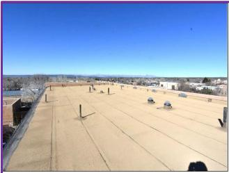
Torch-down roof membrane is in Good Condition and was recently re-roofed, but the edging details will need more work.
