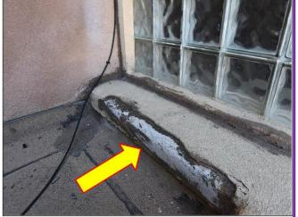
On top of the First story roof deck on the Westside showing damages that are causing leaks underneath the eave and soffit.
