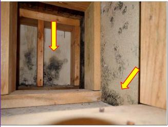
3. Black mold spots found under the Mechanical platform on the walls and sill plate; whereas the drywall will need to be removed for Remediation.
