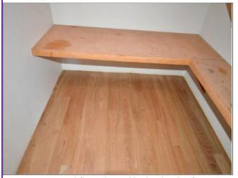
5. Pantry wood floor showed higher levels of moisture under the concrete substrate by 22% that is suspicious.
