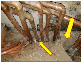
4. Piping through the concrete have holes and are badly cracked and will need to be epoxy sealed to prevent water and moisture from penetrating.
